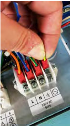
1.18 Replace fan limit stat cables. Yellow to t13 and grey to t15 (plus yellow to t14, brown to t16 and grey to t17 for twin fans) to terminal strip.
