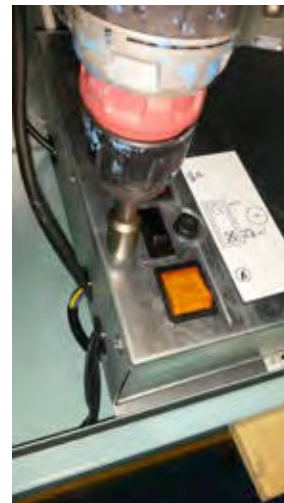
10.23 Replace electrical panel cover.
