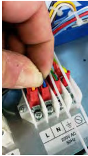
1.16 Replace neutral cable for main fan.
