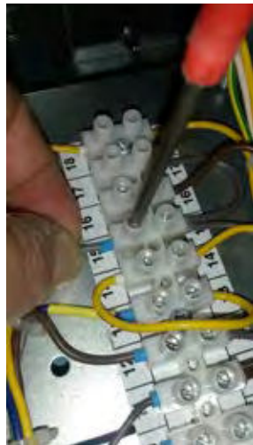
1.18 Replace fan limit stat cables. Yellow to t13 and grey to t15 (plus yellow to t14, brown to t16 and grey to t17 for twin fans) to terminal strip.
