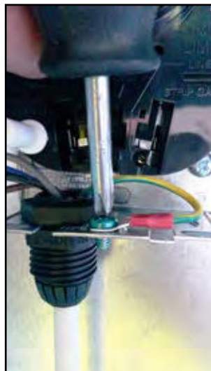
1.3 Remove earth cable - (fork style connector).
