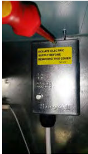
1.5 Remove fixing screw.
