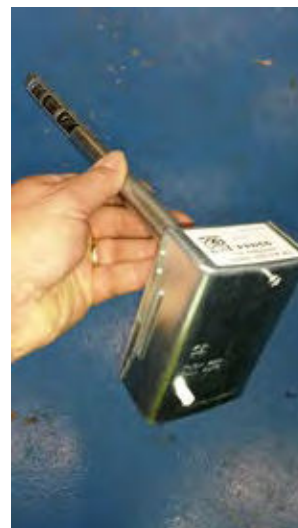
1.8 Locate new stat and remove new cover.
