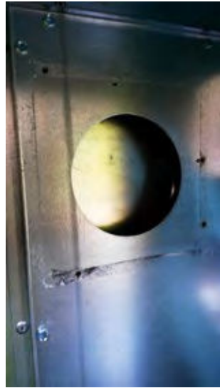
1.9 Exhaust fan removed showing exhaust header plate
