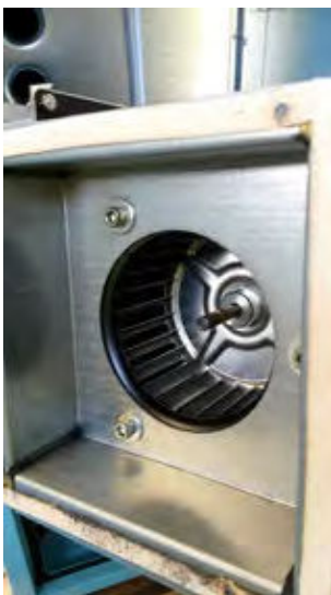
1.11 Place a bead of silicone sealant around the fan inlet. Fit mounting box to new fan using allen head screws. Fit new gasket around flange of mounting box.
