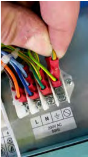
1.17 Refit earth cable to mains block.
